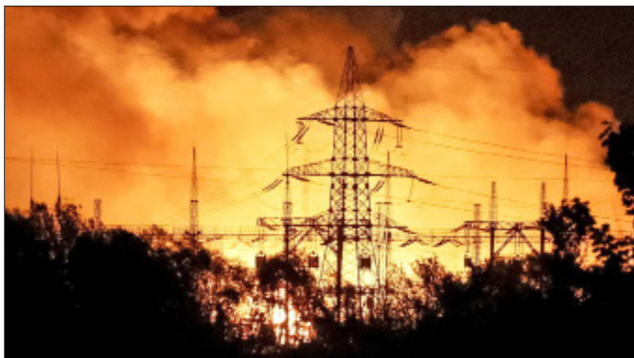
• Ukrainian power plant hit.
